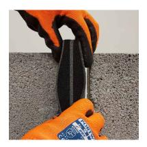
Continue along the length compressing and inserting
