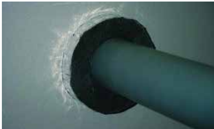
QIF Insulated Fire Sleeve installed in a wall penetration
